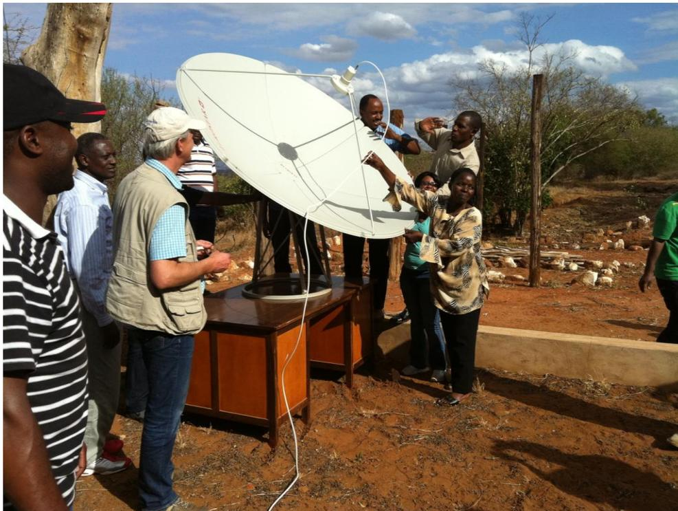
Photo 2 - Pointing of the C-band antenna at the Kenya Wildlife Service Research Station in Voi
